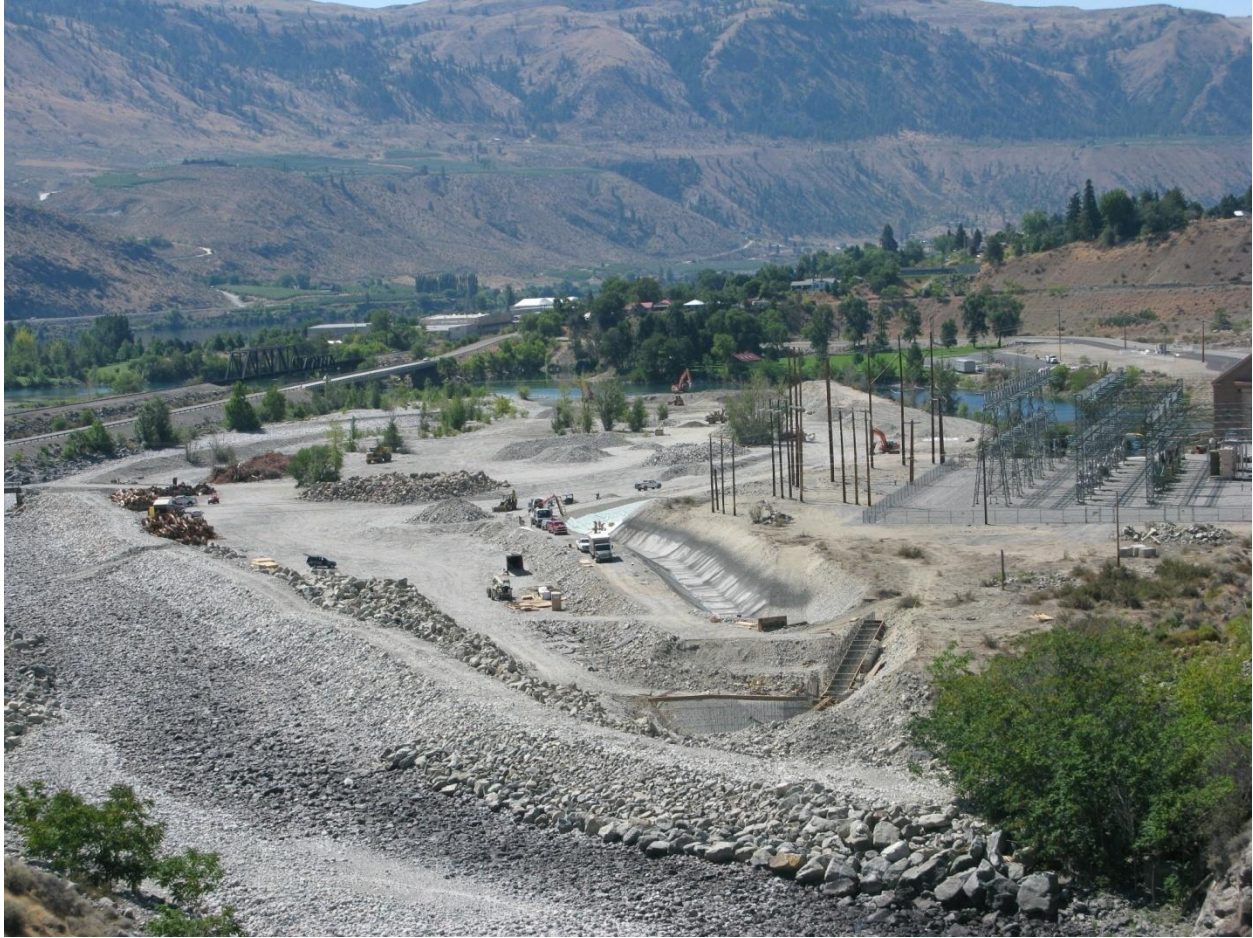
This shows Reach 4 looking south, on August 14 th , 2008. Shotcrete lining of the conveyance canal has begun.
