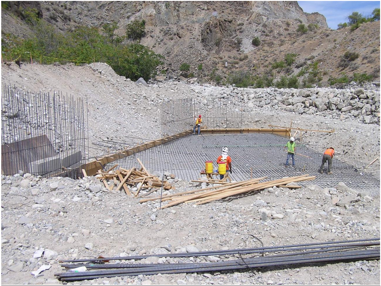
Placement of reinforcing steel and formwork is in progress for the canal outlet structure. August 12, 2008.
