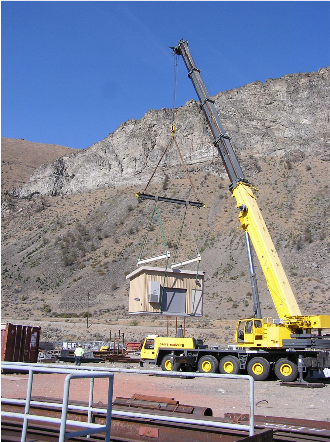
One of two modules of the pump station equipment building is being offloaded. August 15, 2008.
