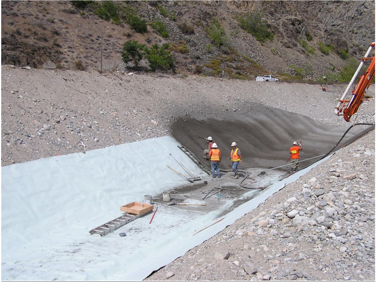
Geo-membrane placement is underway in the canal, and shotcrete placement is beginning. August 12, 2008.
